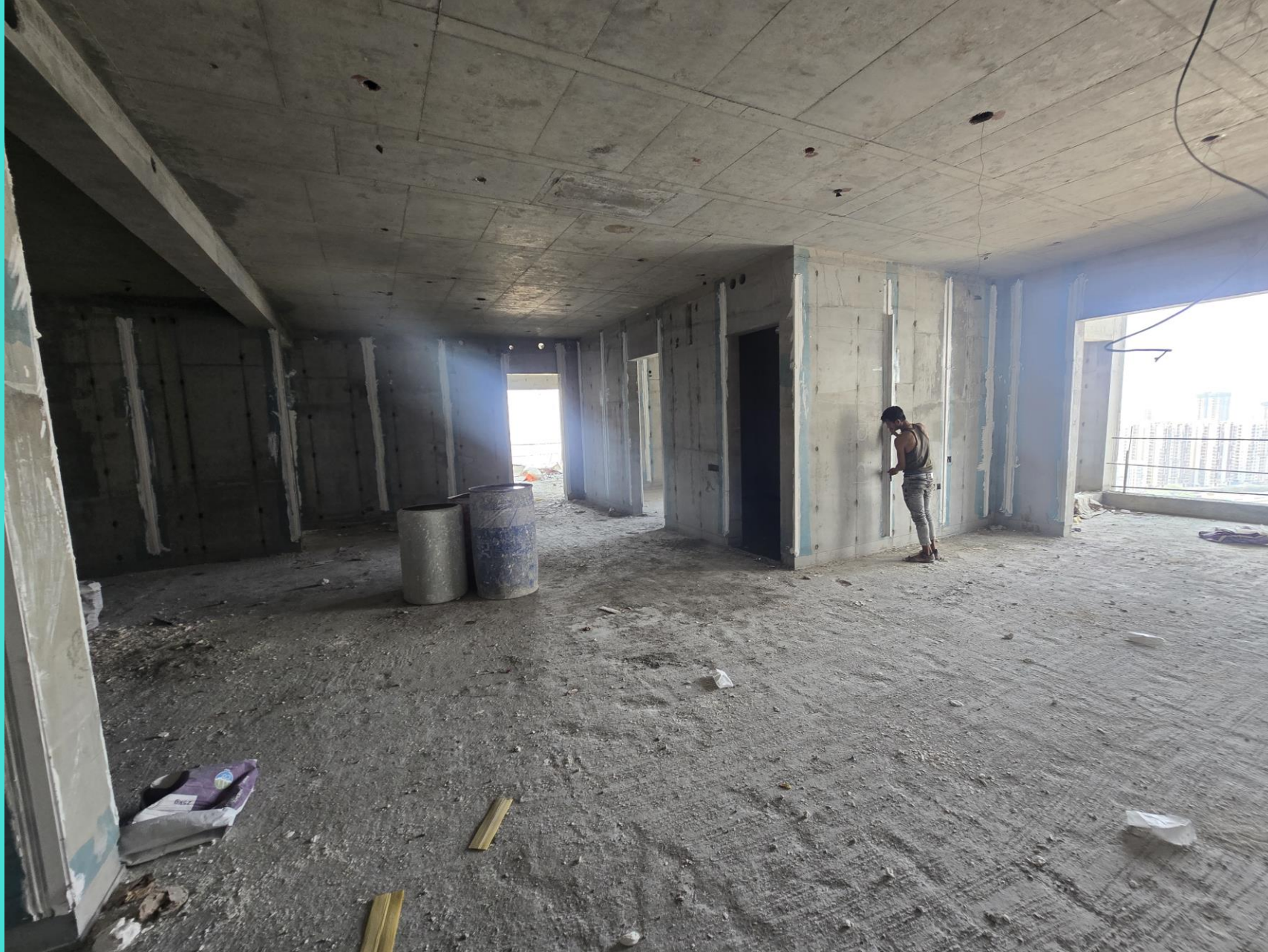
Internal punning level marking.
